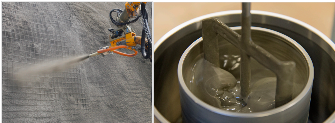
Shotcrete: http://bestsupportunderground.com/rules-for-the-art-of-shotcreting/?lang=en (left), Rheometer testing cement slurry (right)
